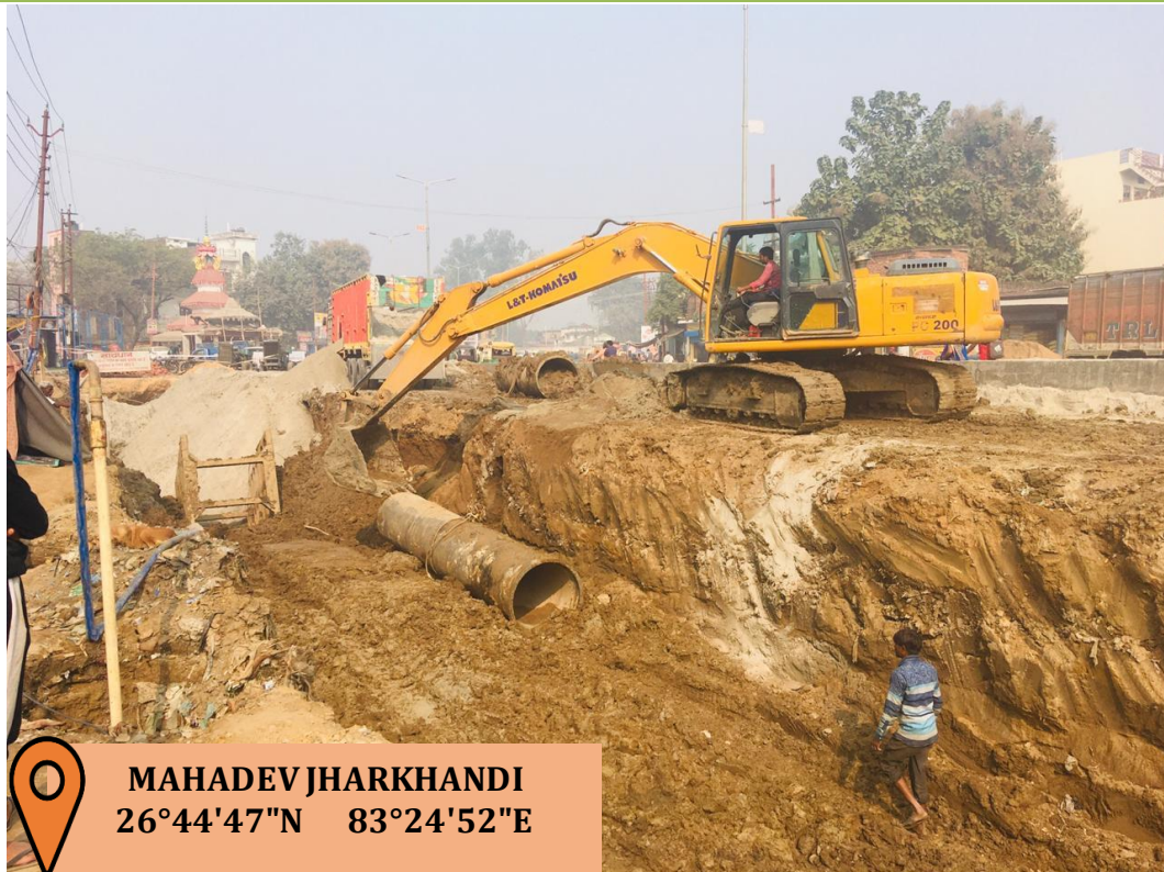
Figure 58: Construction site in Gorakhpur city
